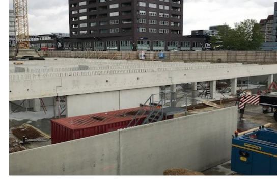
Description Engineering and delivery of columns, beams, floor slabs and
